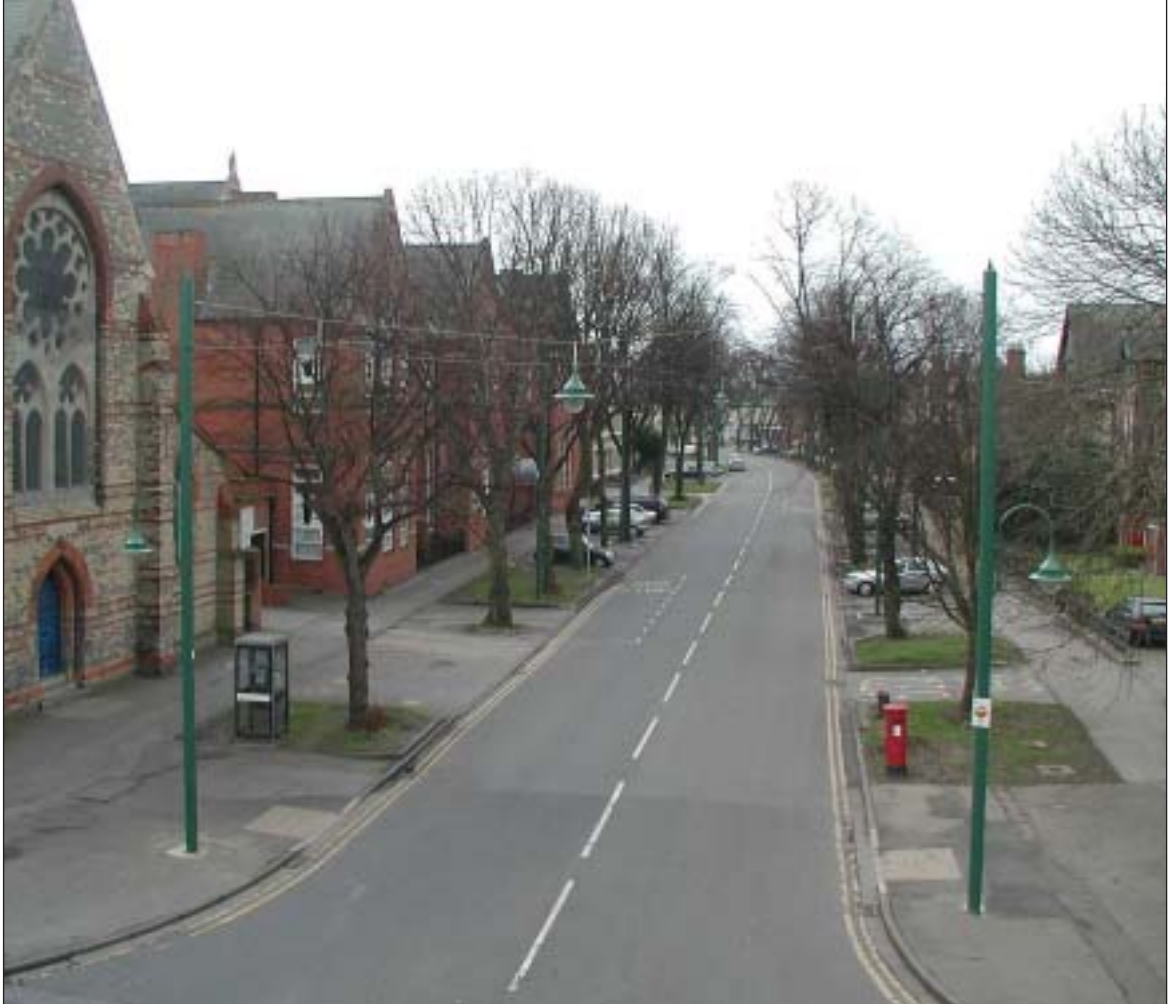
Figure 3.1: The Boulevard, Kingston upon Hull. A lighting scheme designed to light a heavily treed boulevard without extensive pruning of the trees. The carriageway lighting is provided by centrally mounted catenary suspended luminaires using high pressure sodium lamps. The footway lighting is provided by secondary luminaires mounted on the rear of the lighting columns using ceramic metal halide lamps. Photograph by kind permission of Sugg Lighting Ltd.
