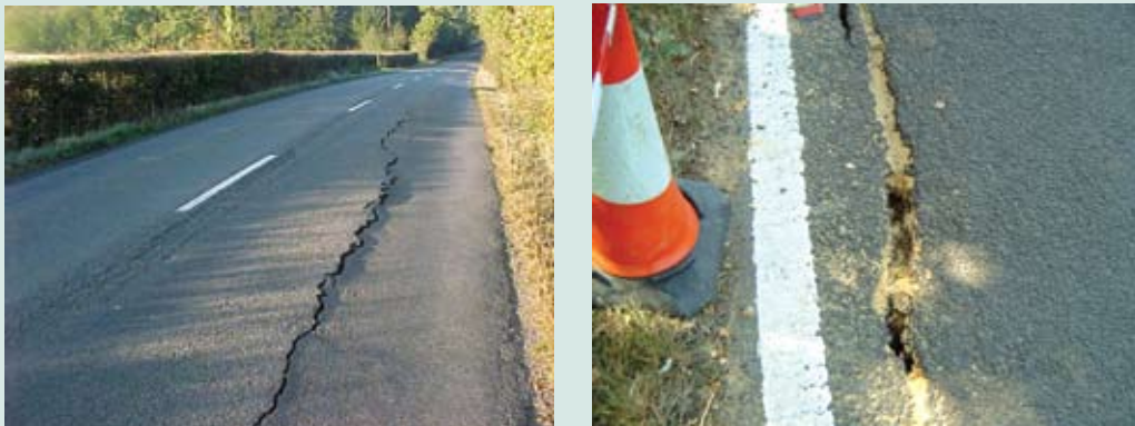
Figure 8.1 Cracking caused by clay shrinkage in Hampshire
