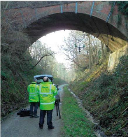
↑ Bridge inspectors fly a drone beneath two very different structures in order to capture condition data and take photographs up close
